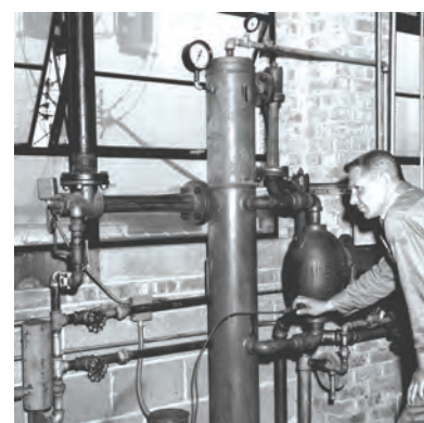
Fig. 28. With available head room at an absolute minimum, S & K engineered this three-stage low-level, condensing unit to eliminate the need for a barometric leg.
