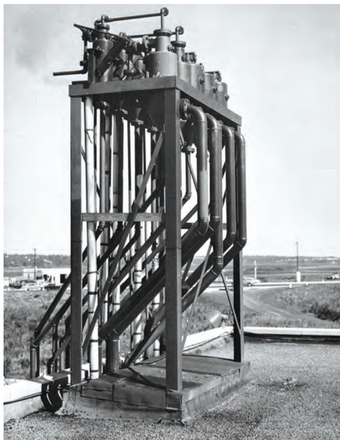
Fig. 18. Five Two-Stage Steam Jet Ejectors equipped with pre-condensers are shown installed on the roof of a chemical plant. Tailpipes on condensers are offset downward at a 45 degree angle to allow free flow of discharge water.
