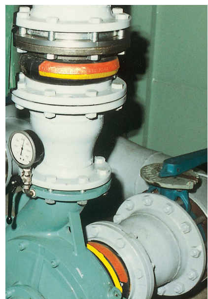
STENFLEX type AR-1 used at pumps
